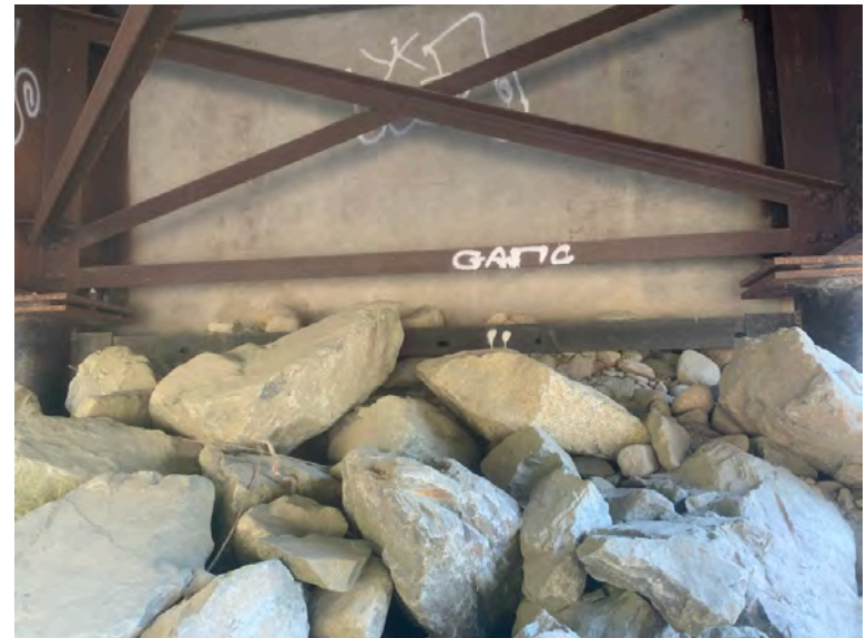
Left Bank Abutment when facing downstream
