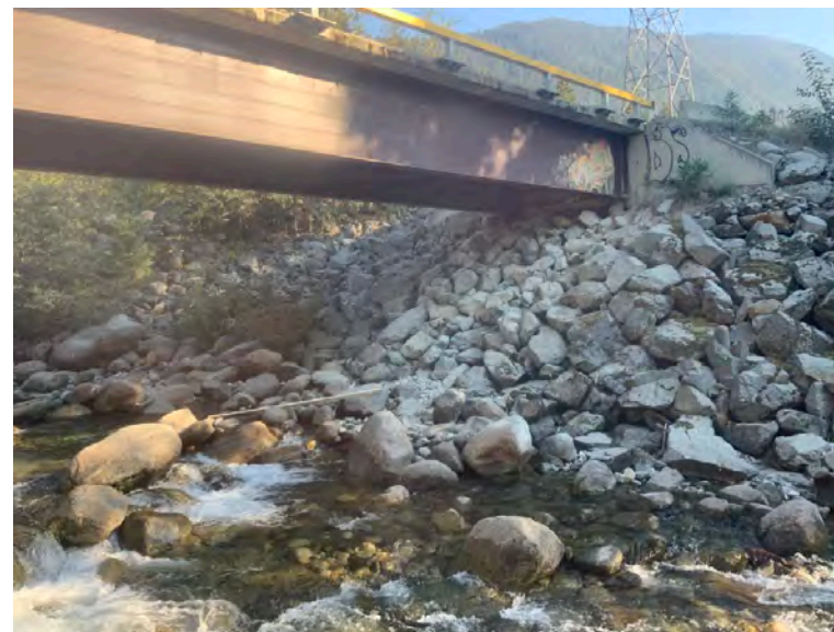
Left Bank Abutment when facing downstream
