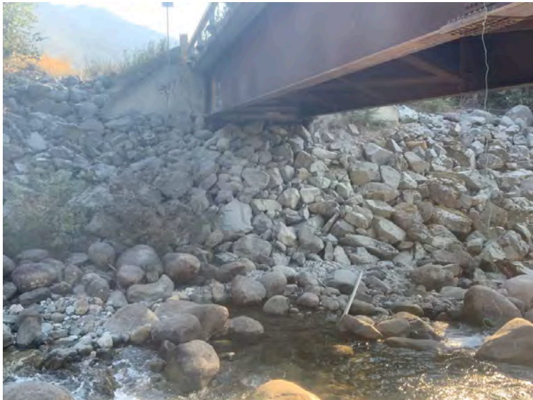
Left Bank Abutment when facing downstream
