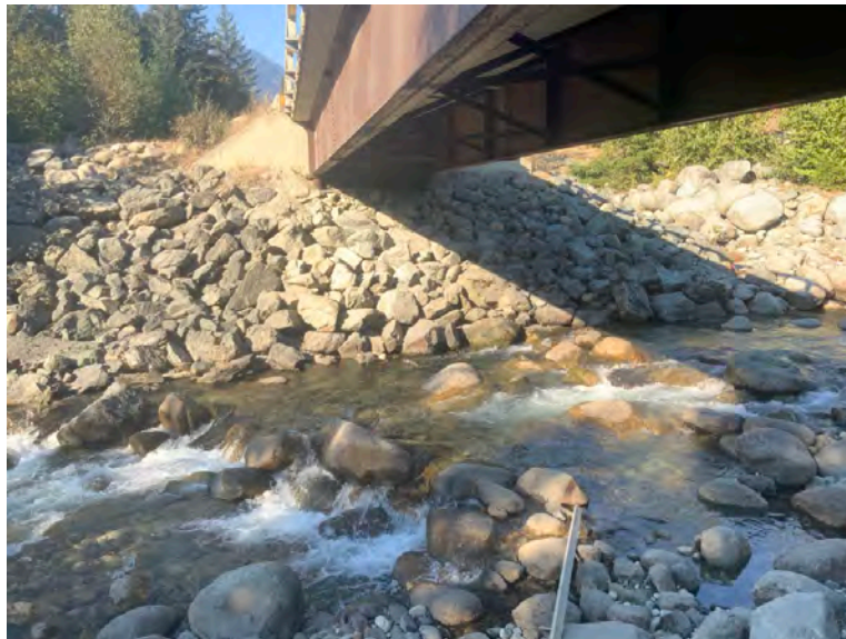
Right Bank Abutment when facing downstream
