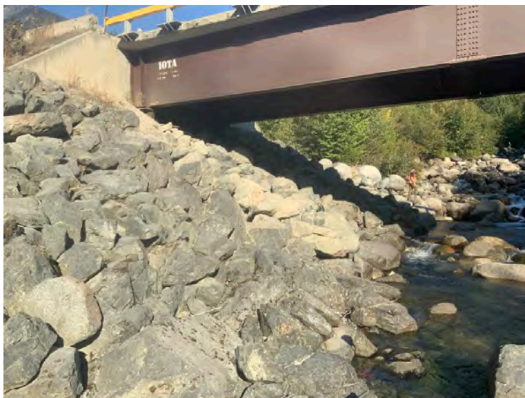
Right Bank Abutment when facing downstream
