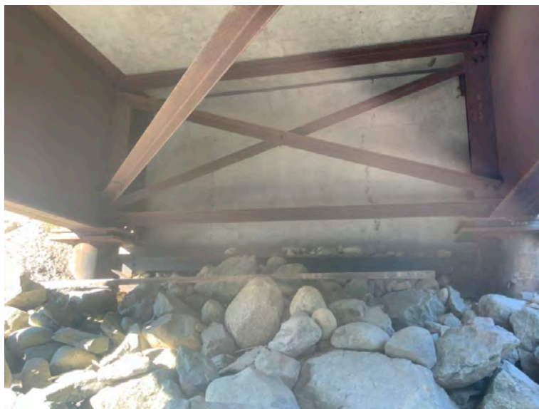
Right Bank Abutment when facing downstream
